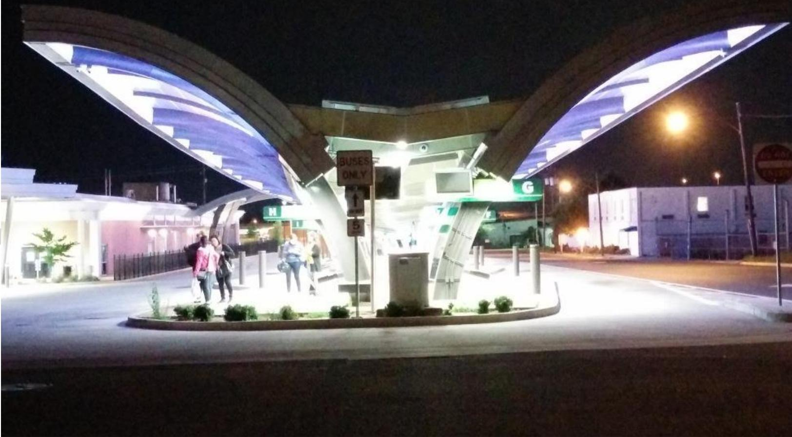
Duo-Gard used its Series 2500 system, engineered for large expanses of sloped glazing. The translucent multiwall polycarbonate in 20mm thickness allows 40% visible light transmittance as it minimizes solar heat gain and glare. The material is shatterproof and completely recyclable.
